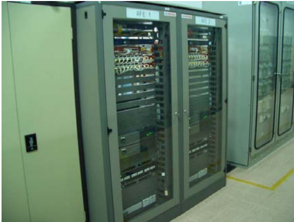
Snapshots: Typical Remote Front End Systems
