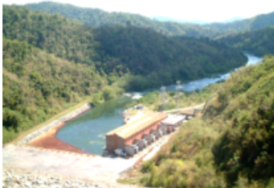
Figure-1: Temengor Station
