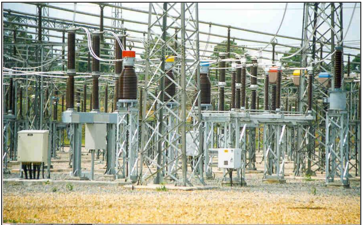
Figure-1: before starting the retro-fitting
